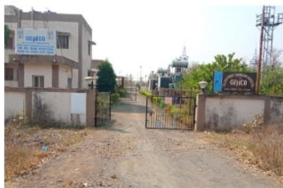
(F-4.4P- Electical power Station)
